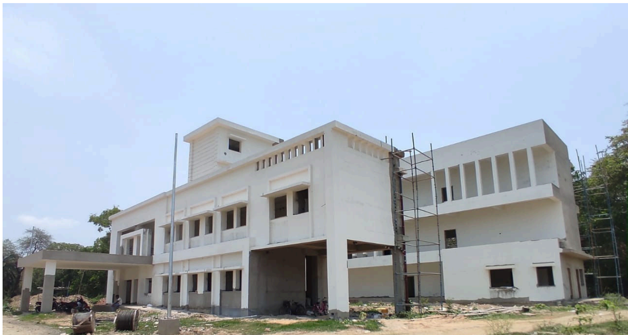
Guest House (Under Construction)
