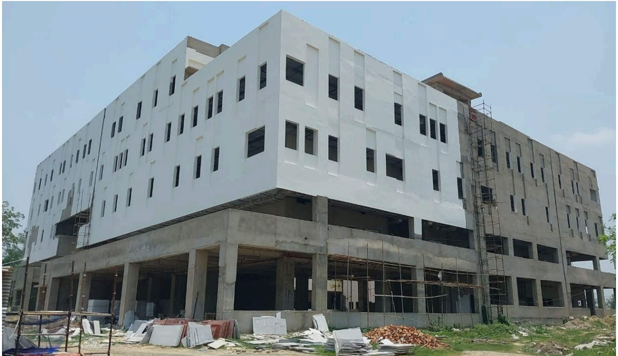
Administrative Block (Under Construction)
