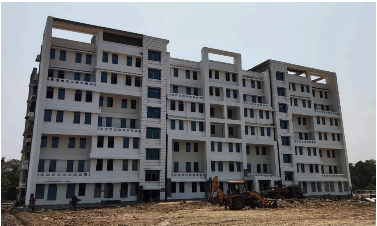
Boys' Hostel (Under Construction)
